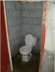
Installation in the Merendón of a pour flush toilet with laundry and shower connected to a soak away septic pit. Toilet flush is done with a small bucket.
